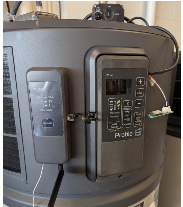
GE water heater with UCM installed and the CTA-2045 port/EcoPort adapter front cover closed.
